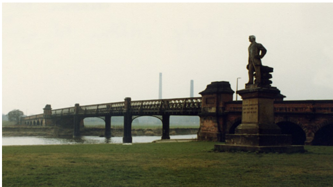
Wilford Toll Bridge (built 1870) and Sir Robert Jukes Clifton.
