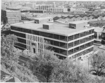
Newcastle House, formerly Viyella House, Castle Boulevard.
